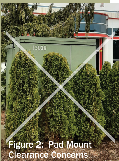
Figure 1: Clearances to Pad Mounted Equipment
